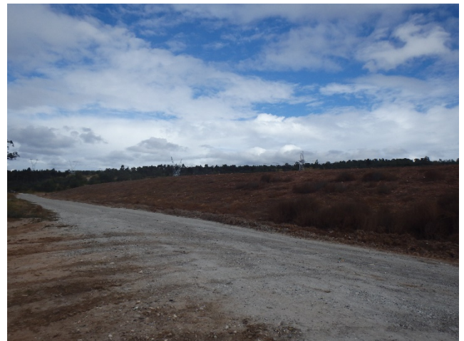
Figure 5 Topsoil stockpile 47, not sown, little vegetation
